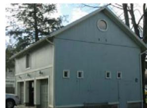
The carriage barn was built prior to 1885 and has hand-hewn mortise and tenon joining, round windows in the gable peak and horse stall windows.
